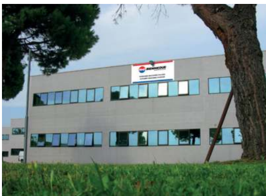
Stabilimento Macchine pulizia Cleaning Division Plant
